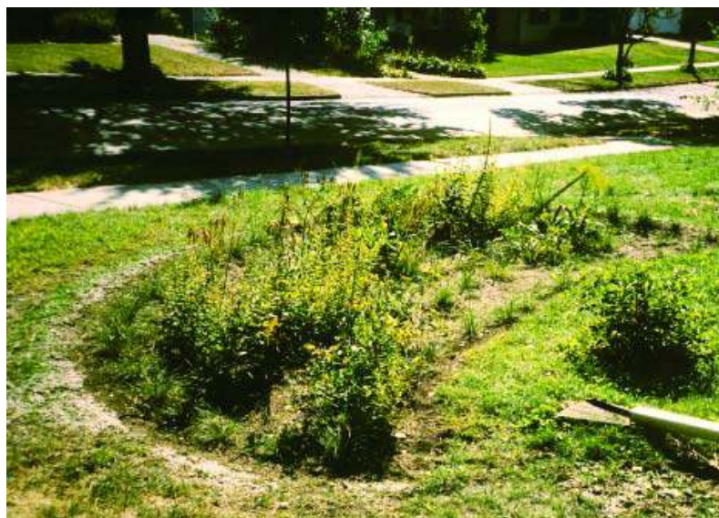
A sample rain garden or bio-retention area.
